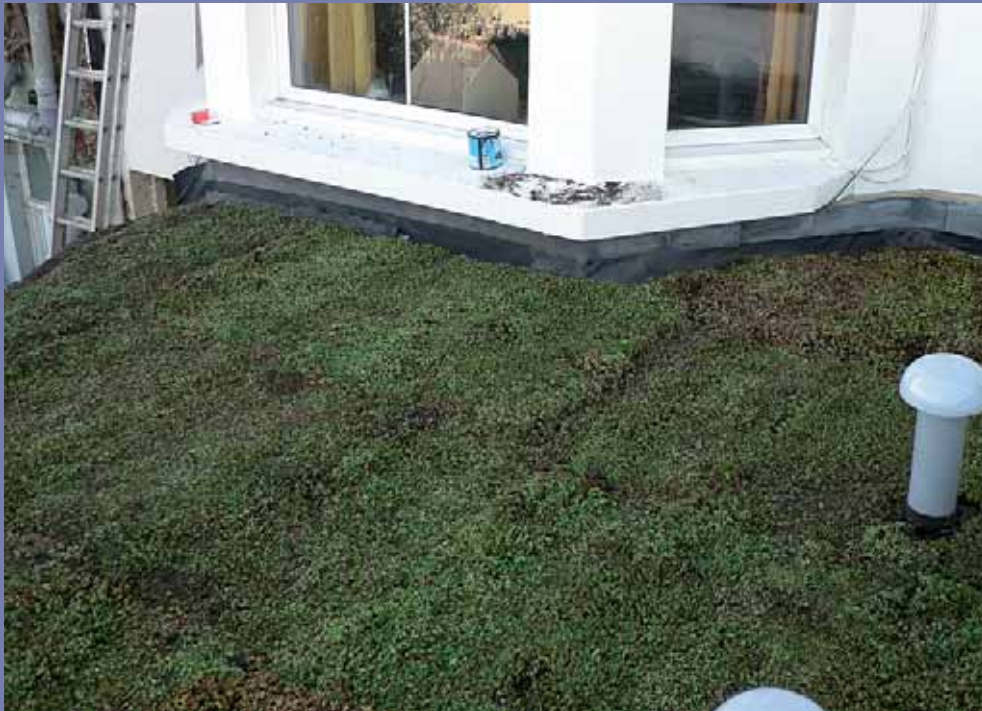
Sedum mat on the roof of an extension. Jeremy Linden
