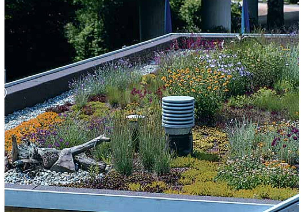
This living roof has been designed to incorporate many different habitats. ZinCo GmbH
