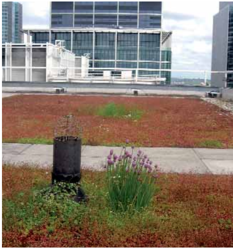
A living roof in Canary Wharf. Dusty Gedge/Livingroofs.org
