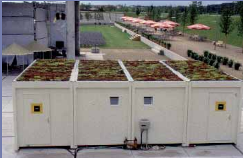
Even Portakabins can be given living roofs. ZinCo GmbH
