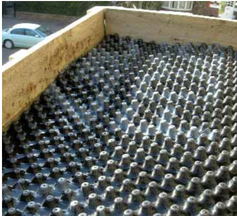
Drainage layer. Dusty Gedge/Livingroofs.org
